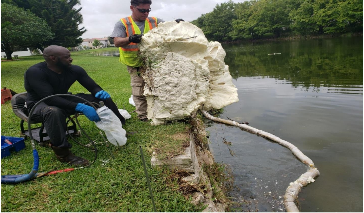
Photo 3: Removal of excessive stabilizing foam resin.
