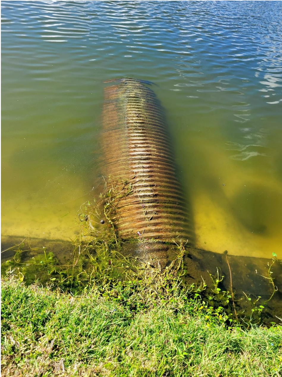
Photo 8: This photo shows the outfall pipe in lake off NW 19 th Court east of NW 74 th Avenue. The pipe is badly corroded and needs to be repaired and/or replaced.
