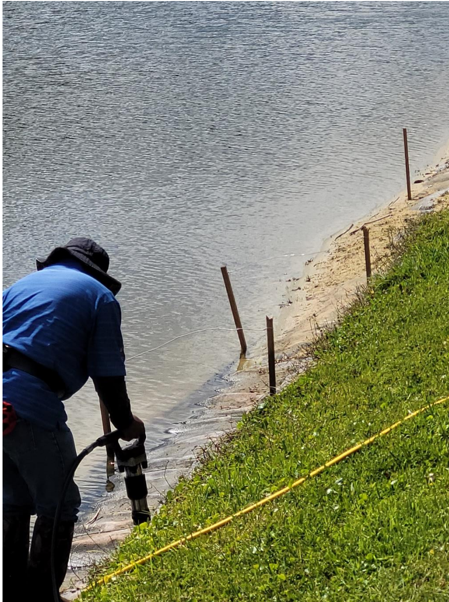
Photo 1: Typical re-attachment of fabric in area of moderate slope. Wire is attached between stakes and an air hammer is used to drive the stakes into the ground near the top and bottom of the exposed fabric.
