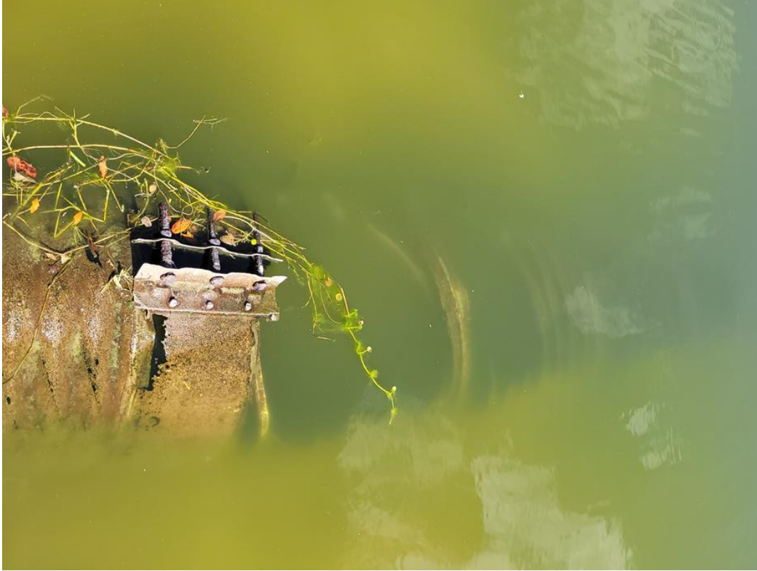
Photo 2: This photo shows the deterioration of the outfall pipe off of NW 16 th Drive. The steel pipe and coupling to the plastic pipe extension has corroded and will need to be replaced. A contractor will need to inspect/televise the pipe between the break and the nearest storm drain and replace the section of corroded pipe.
