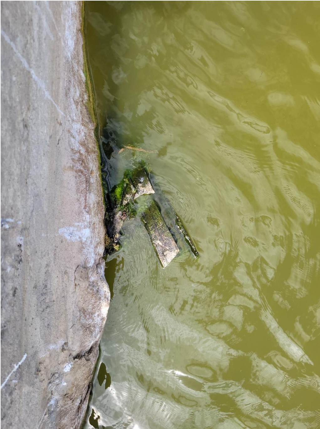
Photo 3: This photo shows the outfall pipe within lake off NW 76 th Terrace as shown in the Special District Services, Inc. report. Investigation shows that the corrugated plastic pipe has been completely broken and the pipe extending out into the lake is missing. The pipe will need to be replaced and should be anchored to prevent this from recurring.
