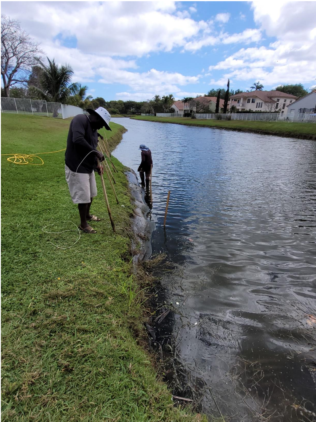
Photo 2: This photo shows a typical installation along a steeper slope. The stakes with attachment wire are closer together (about 3 feet).
