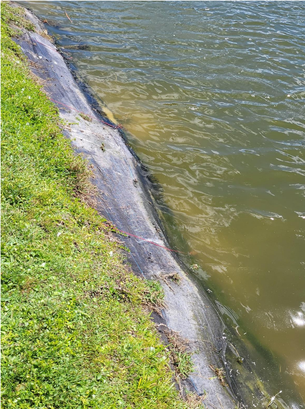
Photo 3: This shows typical completed installation of the attachment. Note the red wires are visible on top of fabric between the stakes that are not clearly visible.
