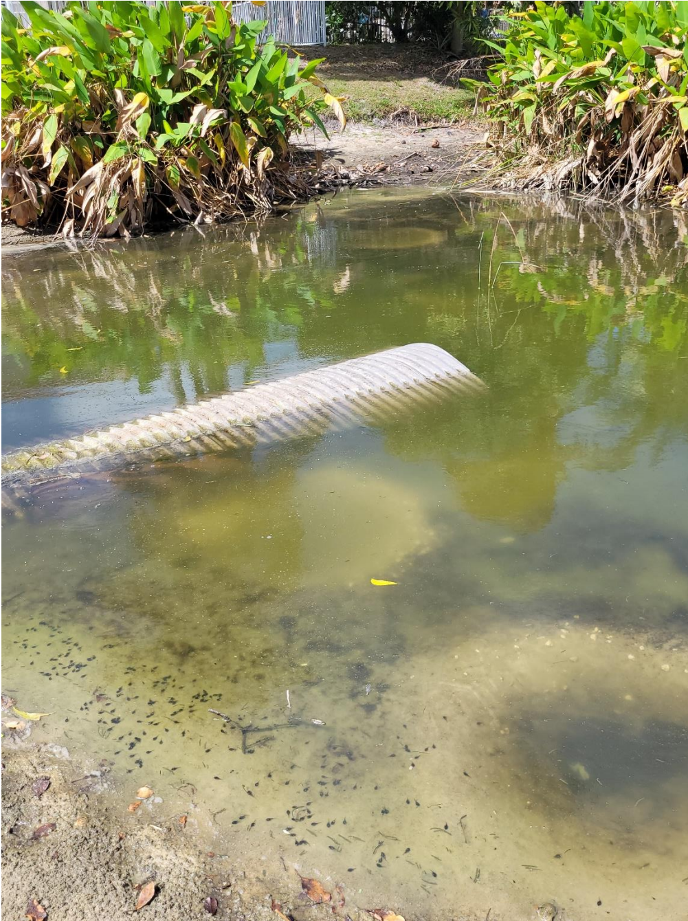
Photo 5: This photo shows the outfall pipe in lake off NW 20 th Street. The pipe has 6 inches of sediment requires cleaning. In addition, the outfall pipe may require extending and sediment may need to be removed from the lake bank surrounding the outfall and the line extended to a deeper location within the lake.
