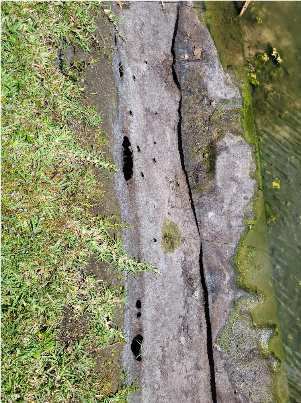
Photo 4: This photo shows section of fabric that is starting to decay due to continuous exposure to the sun. Once the material has been compromised, animals, such as Iguana, can expand these holes to make underground burrows.
