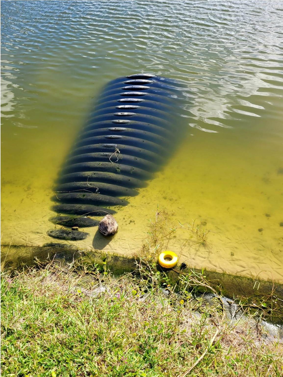
Photo 9: This photo shows the outfall pipe in lake off NW 74 th Avenue south of NW 19 th Court. The pipe has severe sediment buildup and needs to be cleaned, extended into lake and/or lake sediment removal by means of dredging.
