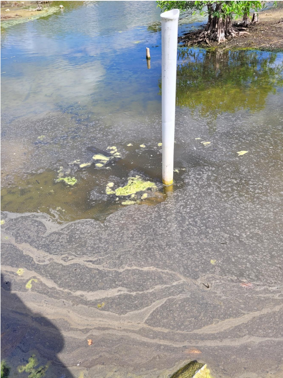
Photo 7: This photo shows the outfall pipe in lake off NW 78 th Way. The pipe has 12 inches of sediment. The outfall needs to be cleaned, extended into lake and/or lake sediment removal by means of dredging.
