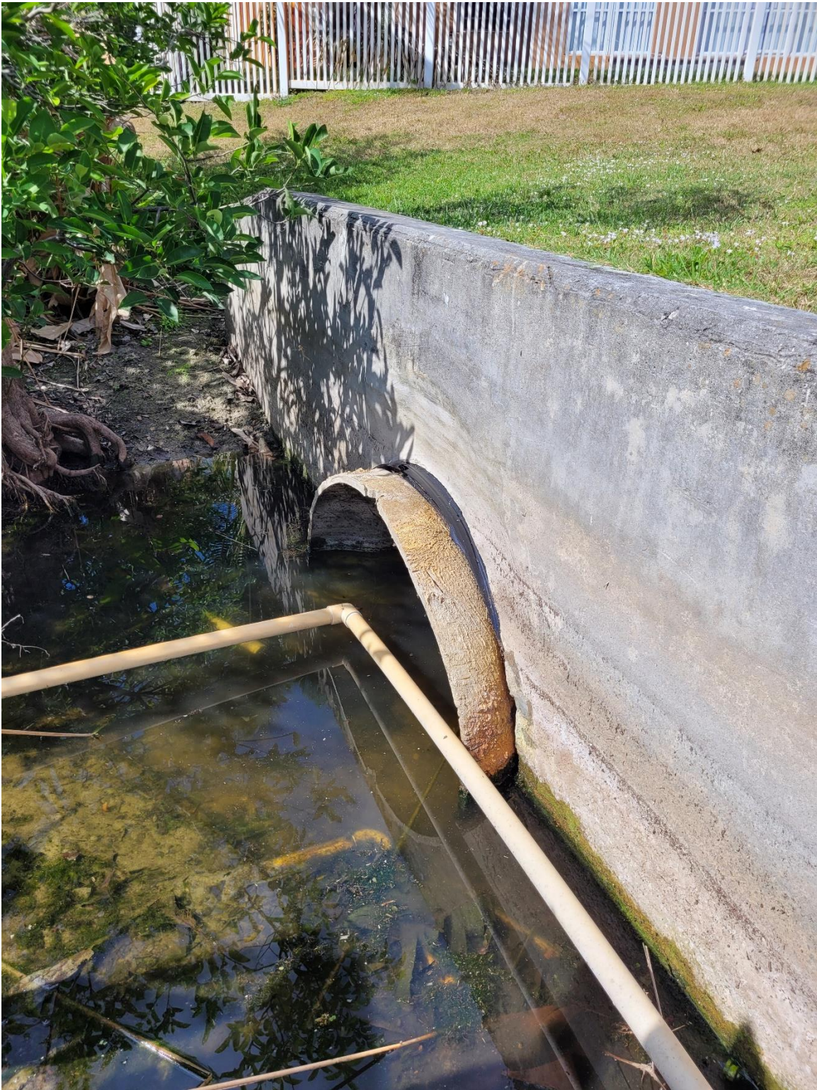
Photo 6: This photo shows the outfall pipe in lake off NW 19 th Court. The pipe has 12 inches of sediment buildup. The outfall pipe needs to be cleaned with a pipe extension into the lake and/or lake sediment removal by means of dredging.
