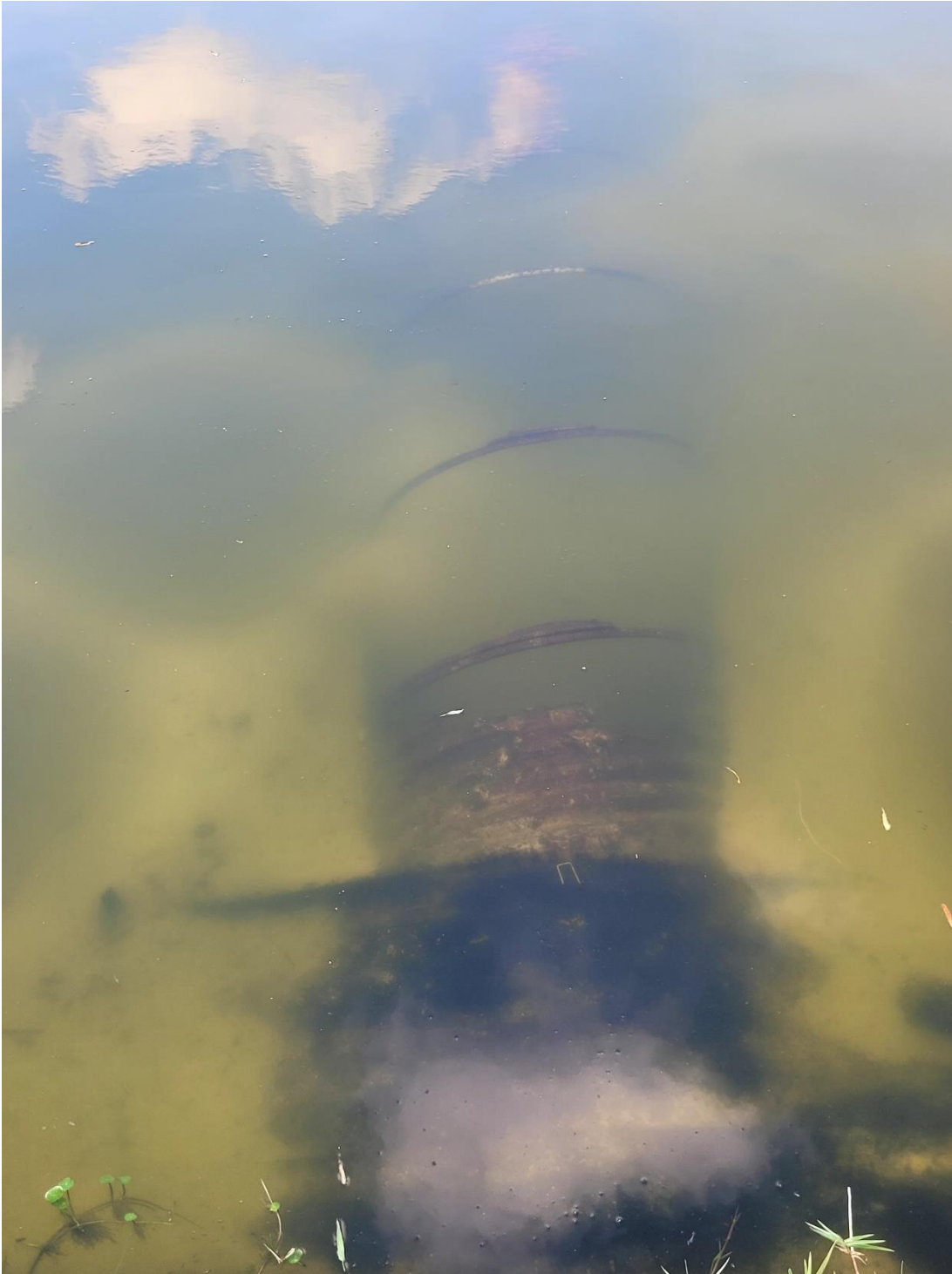
Photo 10: This photo shows the outfall pipe in lake off NW 72nd Way north of NW 18 th Court. The outfall pipe has completely corroded away and needs to be replaced. The pipe needs to be cleaned and inspected/televised back to the nearest catch basin in the road to determine the condition of the entire pipe. This pipe may collapse if not repaired.
