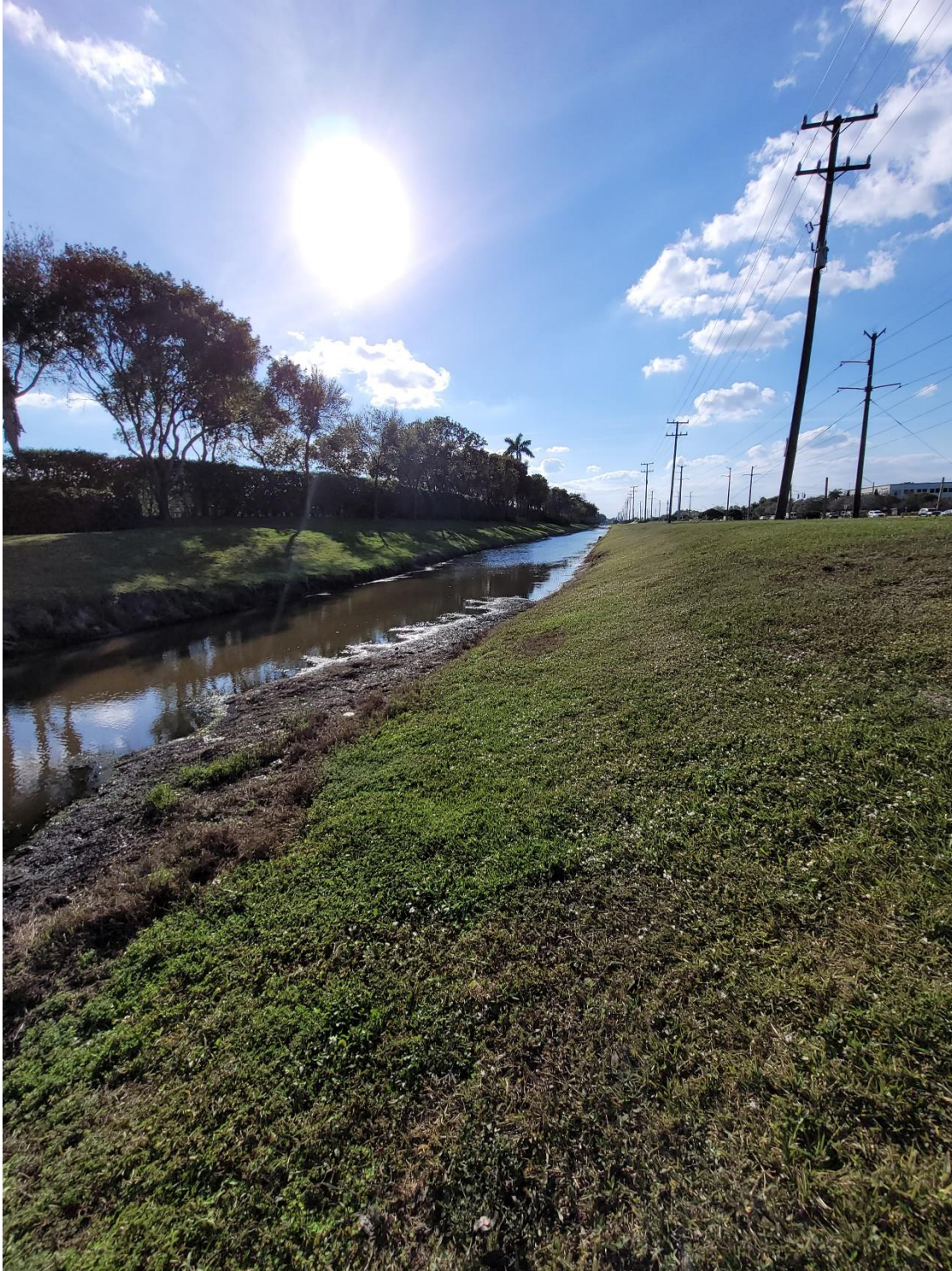
Photo 4: East/west canal parallel to Sheridan Street and west of NW 72 nd Avenue, looking west. The photo indicates sediment build up along the north bank of the canal, within the scope of the NW 72 nd Avenue canal restoration project.
