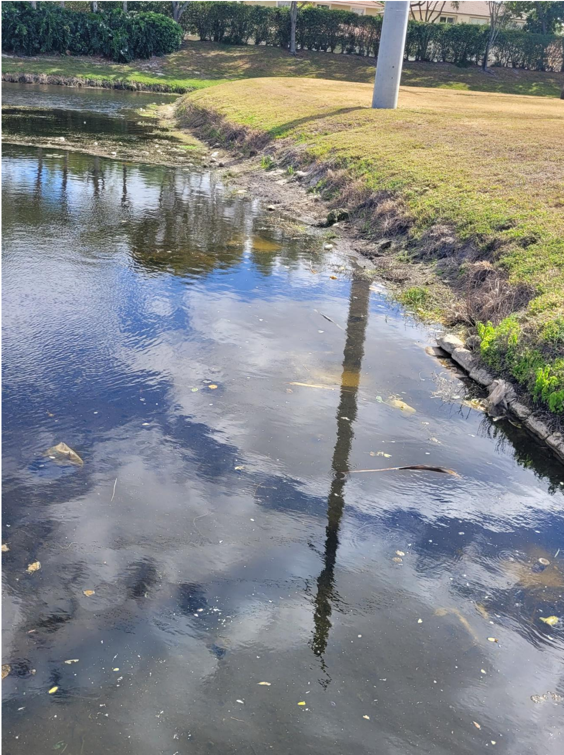
Photo 6: West bank of canal section at Sheridan Street and the 7300 block, looking south. The photo indicates the erosion of approx. 135-feet of the west bank.
