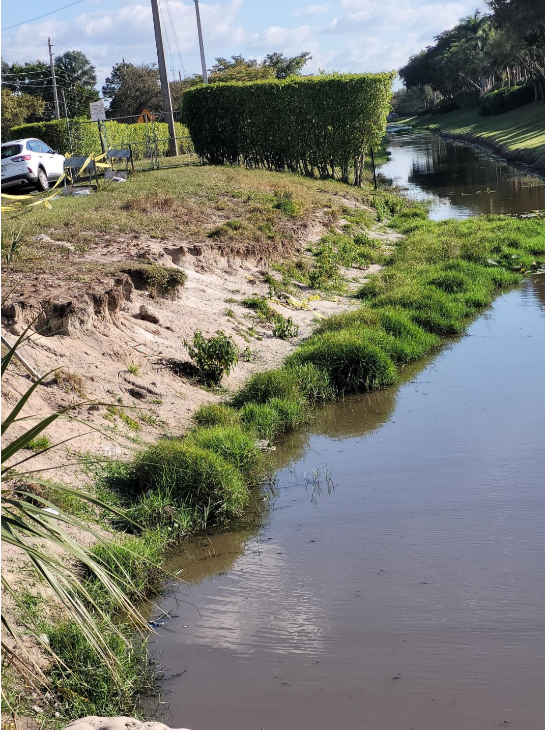
Photo 2: The east side of the canal bank adjacent to NW 72 nd Avenue, looking south. The photo indicates the approx. 135-feet of washed out sugar sand.
