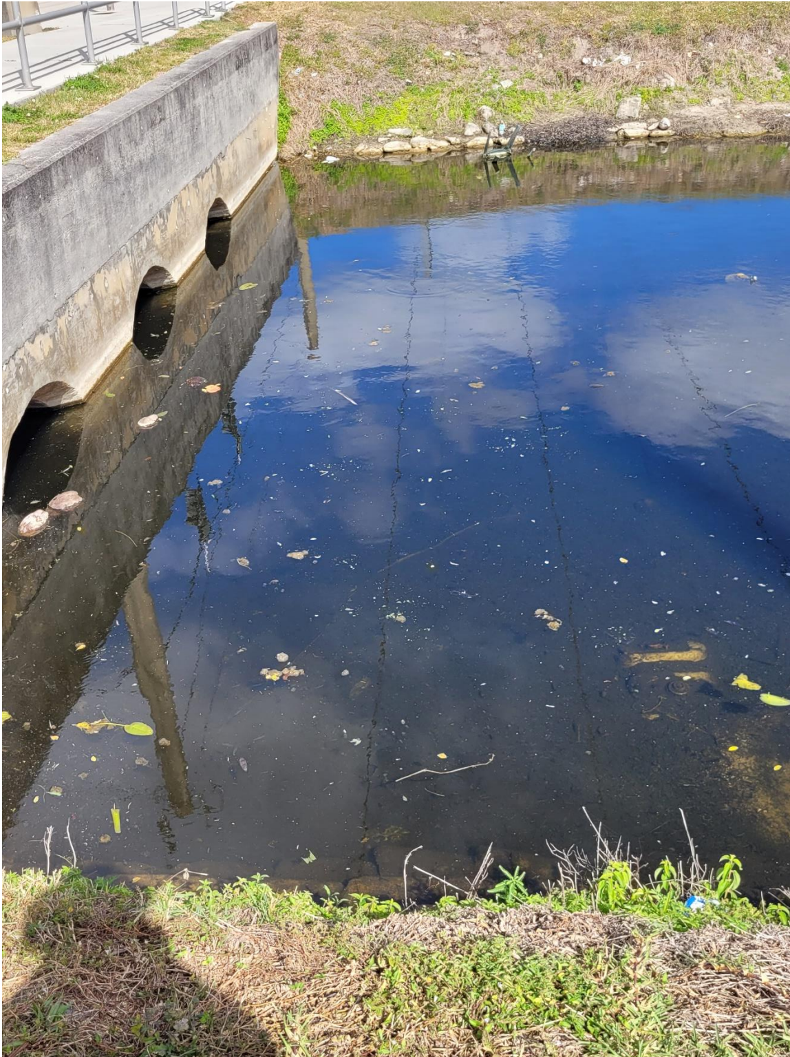
Photo 5: North side of canal section at Sheridan Street and the 7300 block, looking east. The photo shows the three culverts on the south side of Sheridan Street and that the sediment build-up in half of the pipe and all but 6-inches in the canal has greatly impeded flows.
