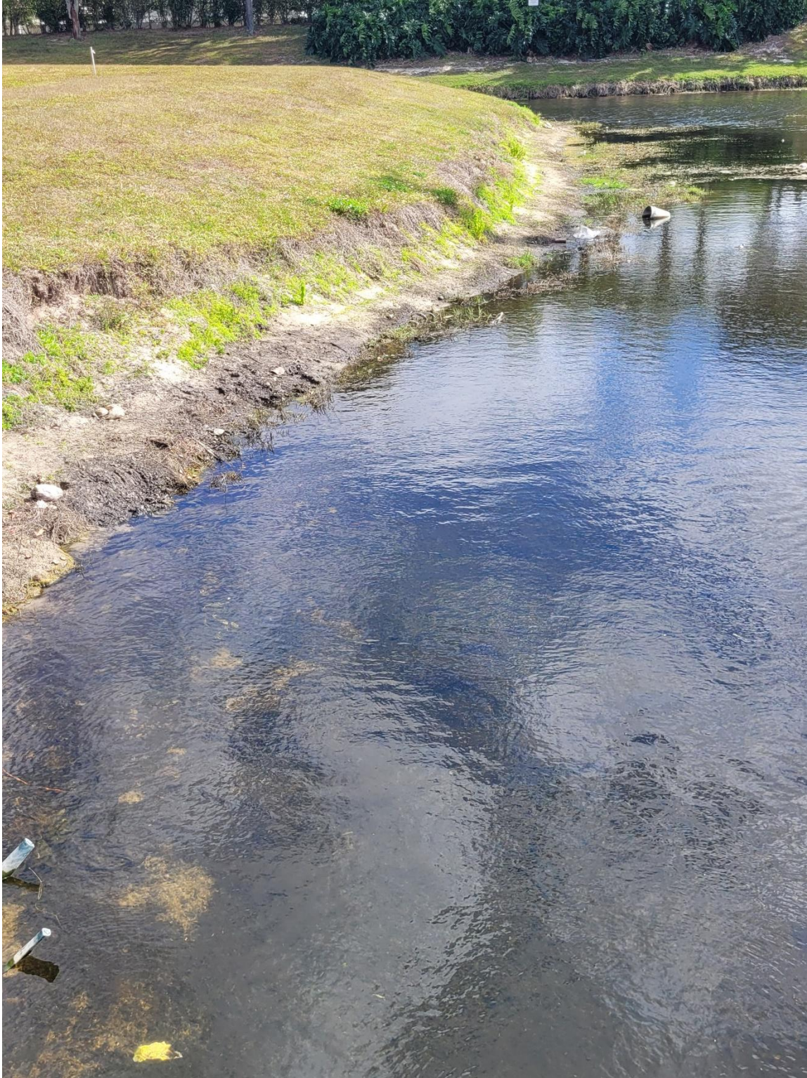
Photo 7: East bank of canal section at Sheridan Street and the 7300 block, looking south. The photo indicates the erosion of approx. 150-feet of the east bank.
