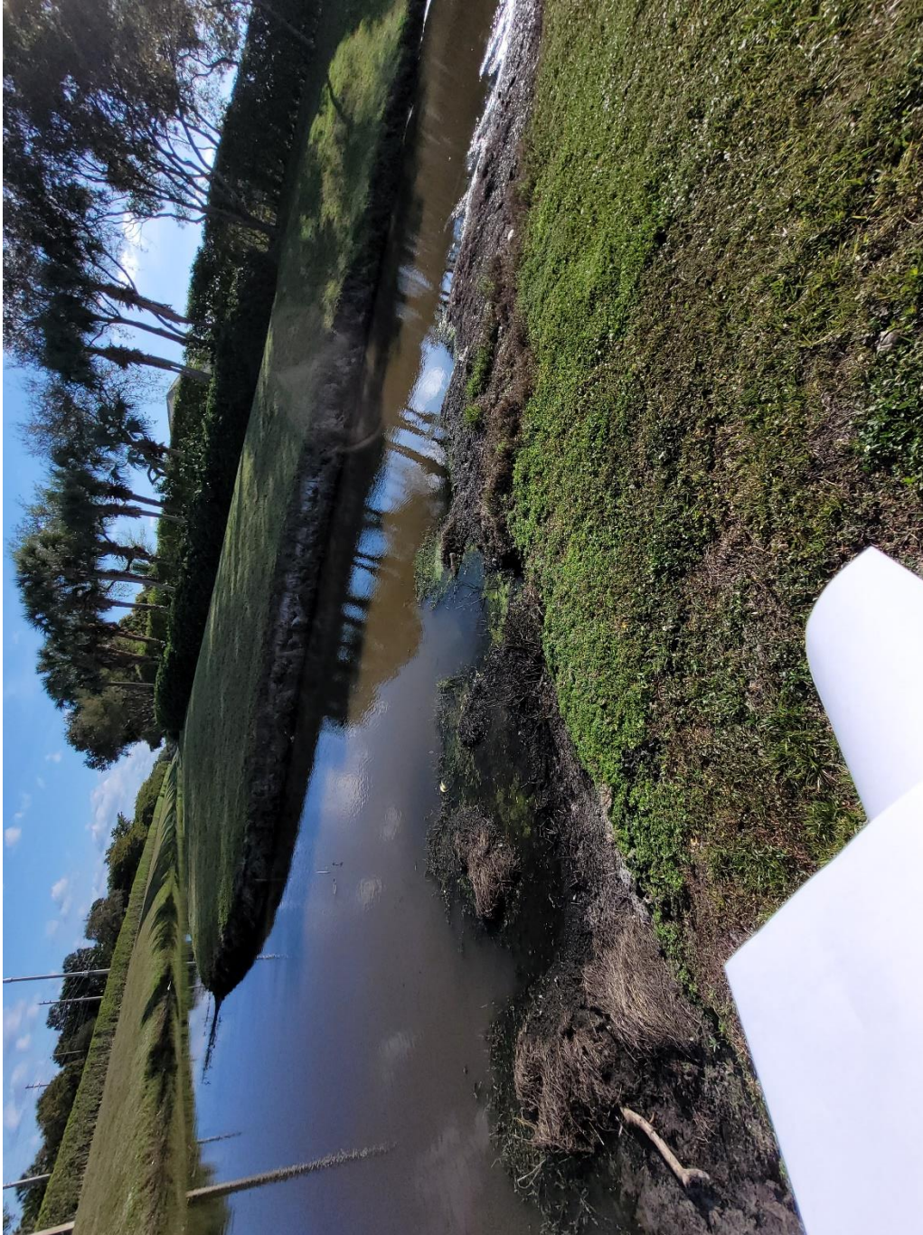
Photo 3: NW 72 nd Avenue canal section, looking south. The photo indicates the bank erosion and silt build up at the canal intersection.
