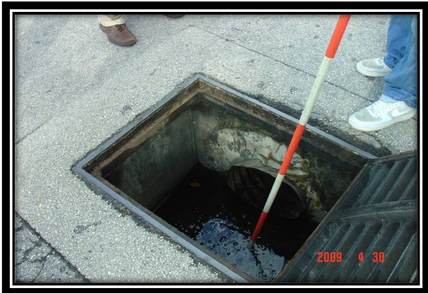
Missing Pollution Retardant Baffles
