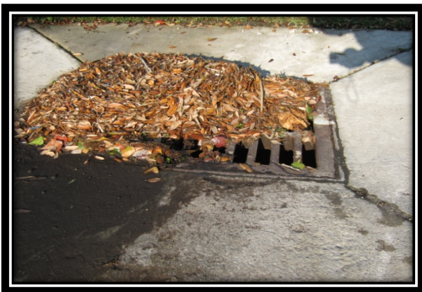
Storm Drain Blockage
