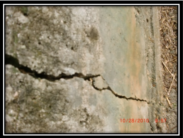
Headwall Cracks
