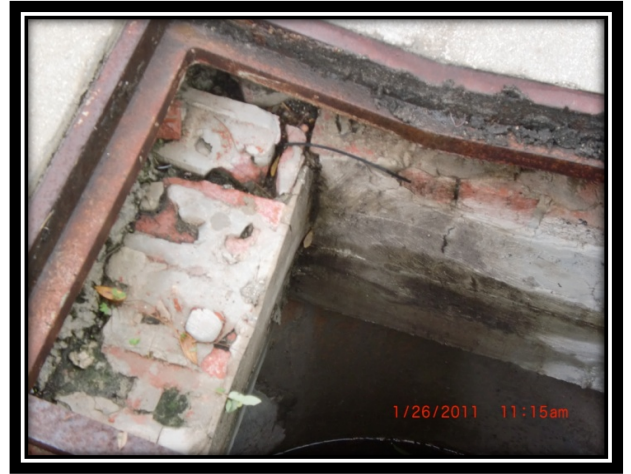
Concrete Repairs Required Inside Catch Basin
