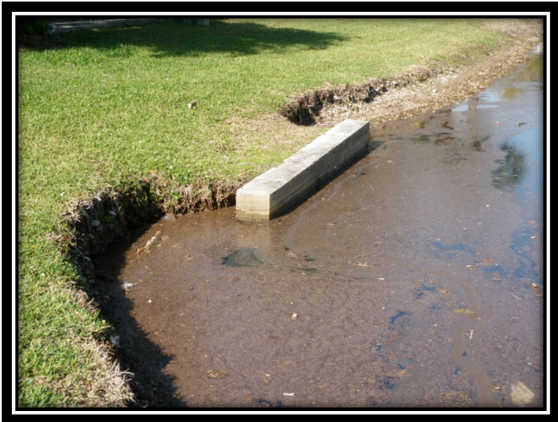
Headwall Erosion
