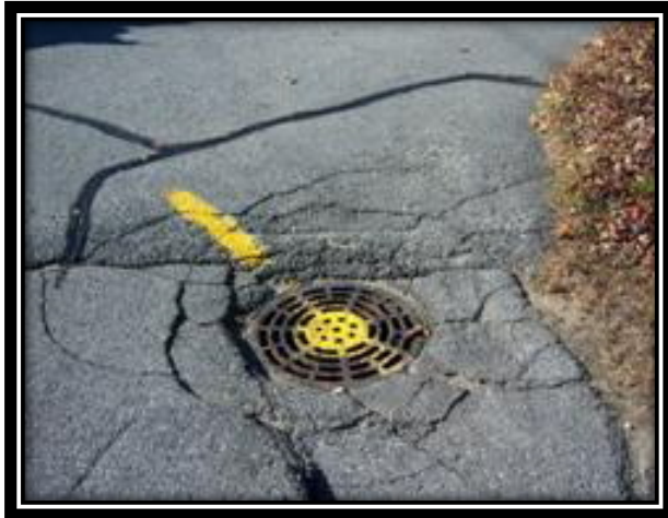
Asphalt Deterioration
