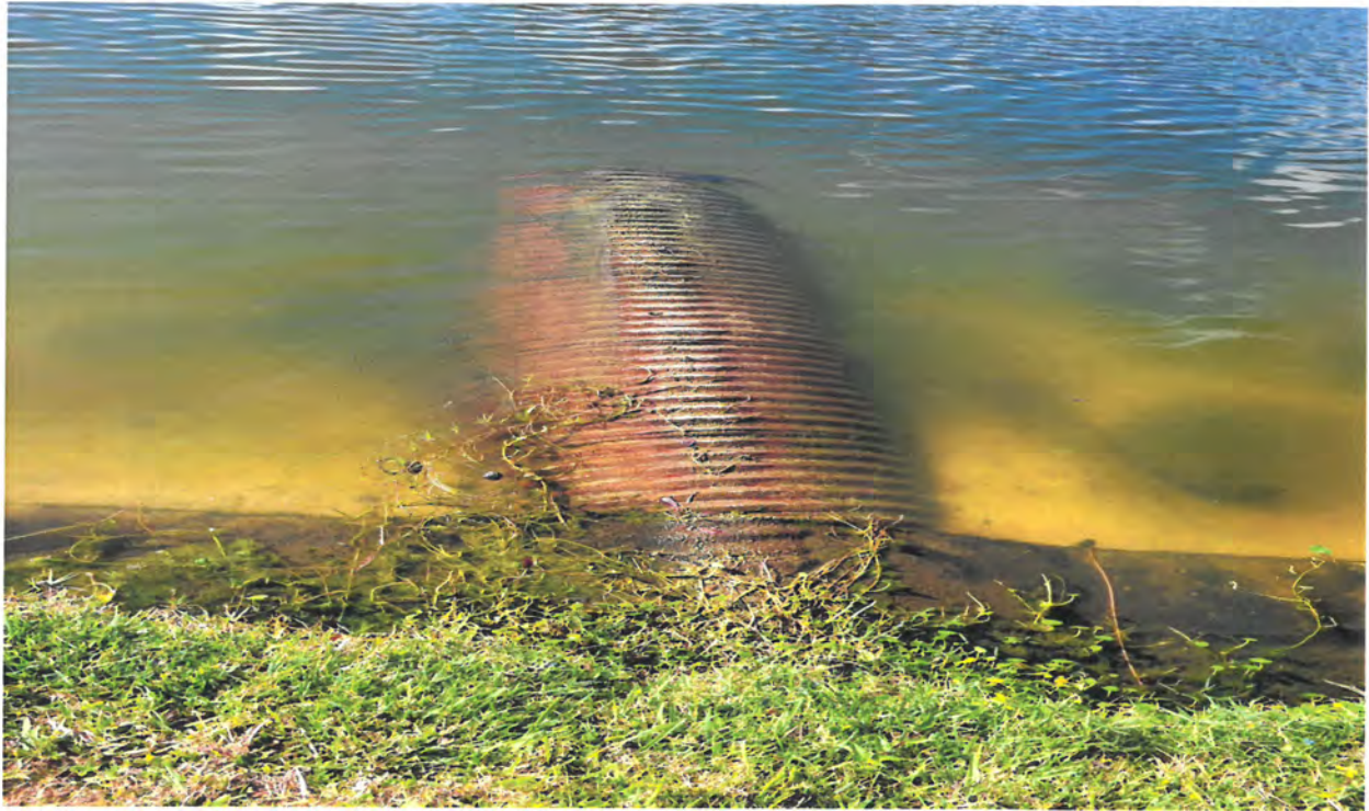
Photo 9: Corroded outfall pipe at Lake 4 (near NW 19 Court) during inspection in March, 2023.
