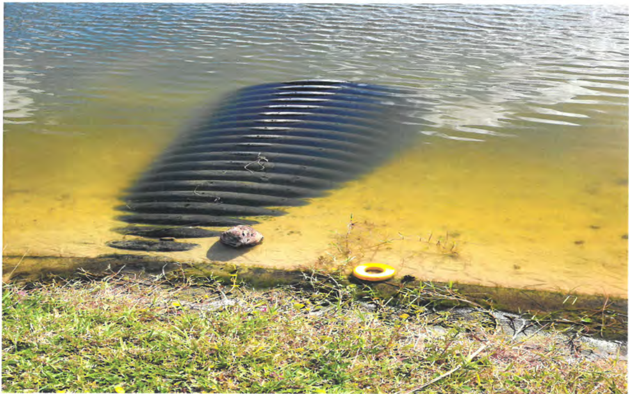
Photo 10: Sediment buildup at outfall pipe at NW 74 Ave in Lake 4 during inspection in March, 2023.
