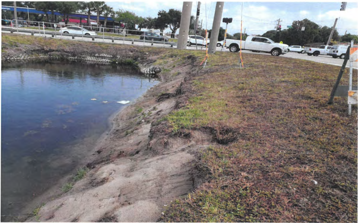
Photo 1: Culvert and canal bank erosion at Sheridan Street and N 72 Avenue.
