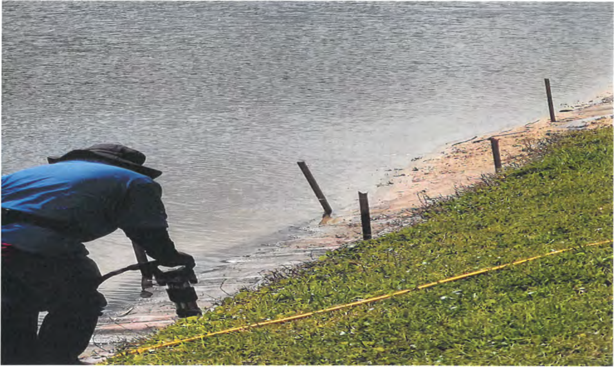
Photo 7: Anchoring of fabric material at lake banks by American Shoreline in March, 2023.
