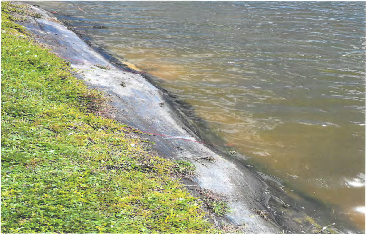
Photo 8: Completed re-installation of lake bank fabric material.
