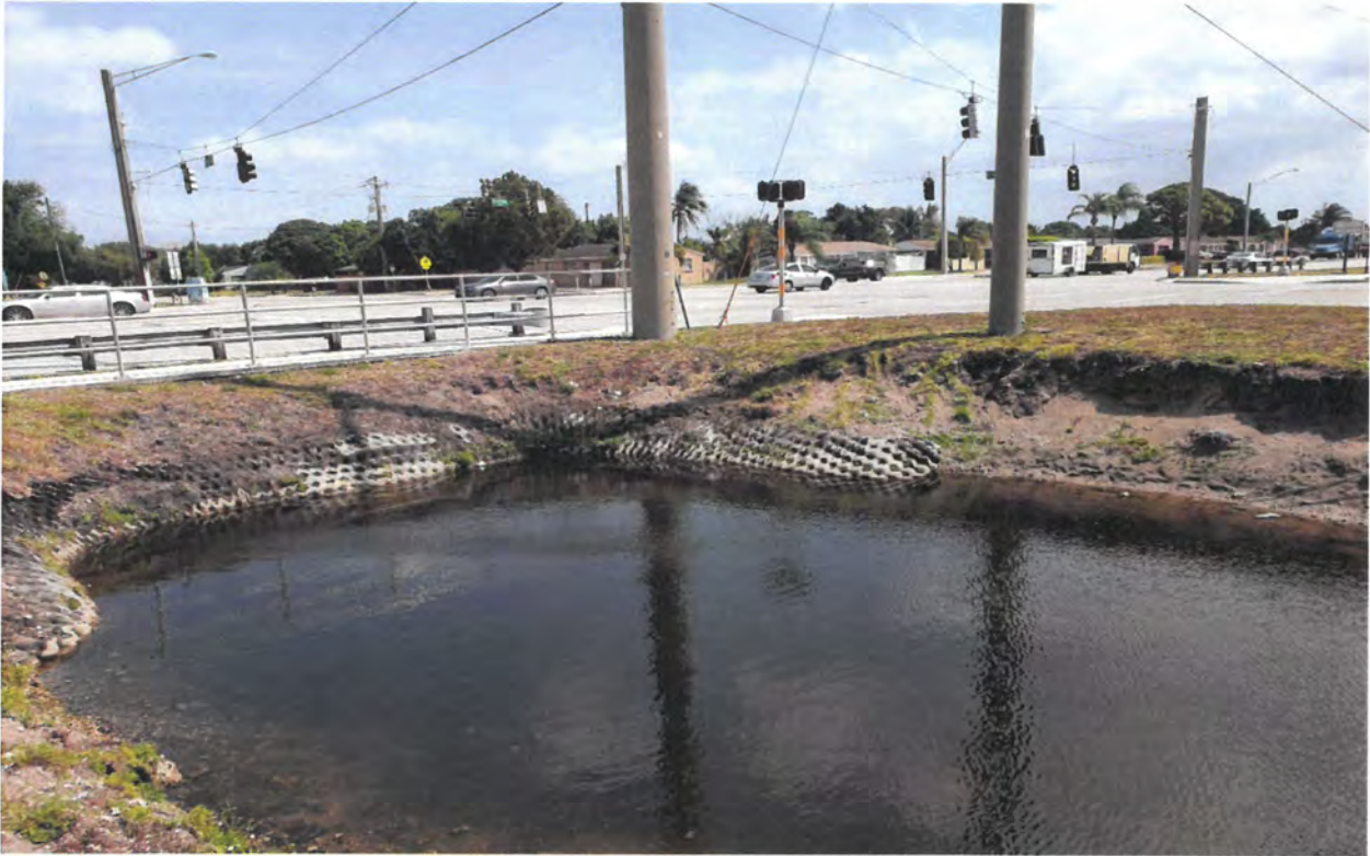
Photo 3: Culvert and canal bank erosion at Sheridan Street and N 72 Avenue.
