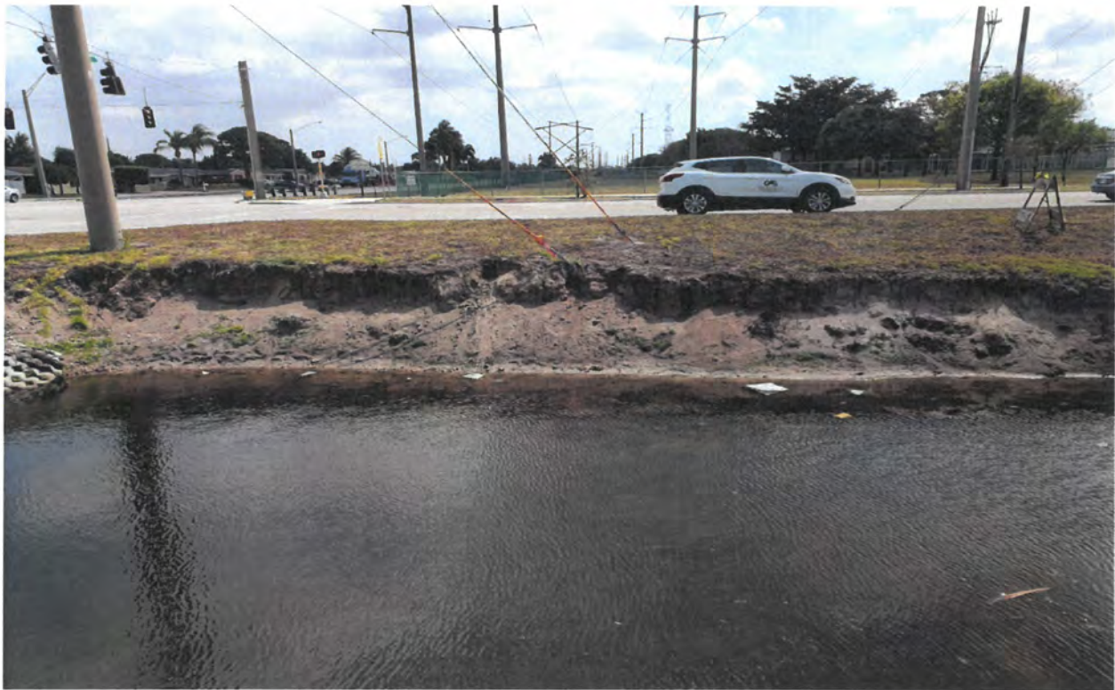
Photo 2: Culvert and canal bank erosion at Sheridan Street and N 72 Avenue.
