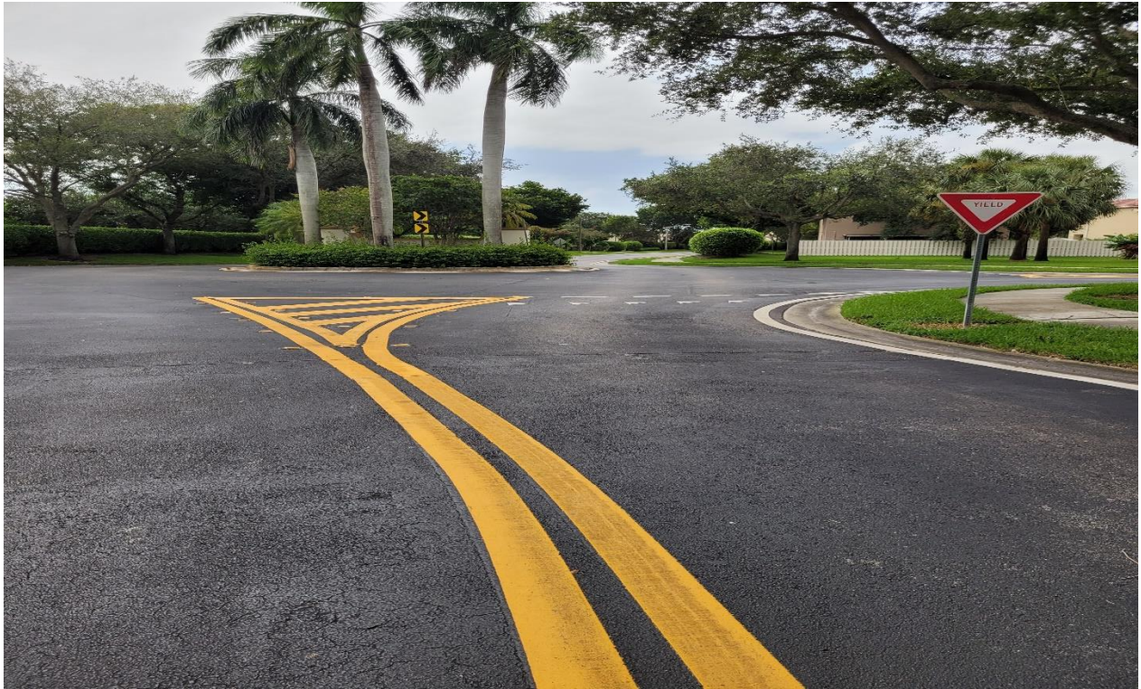
Photo 5: Sealcoating and restriping of internal WCCDD roads performed in 2022.
