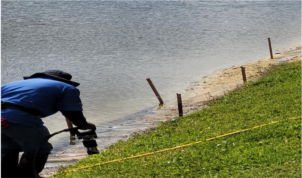
Photo 7: Anchoring of fabric material at lake banks by American Shoreline in March, 2023.
