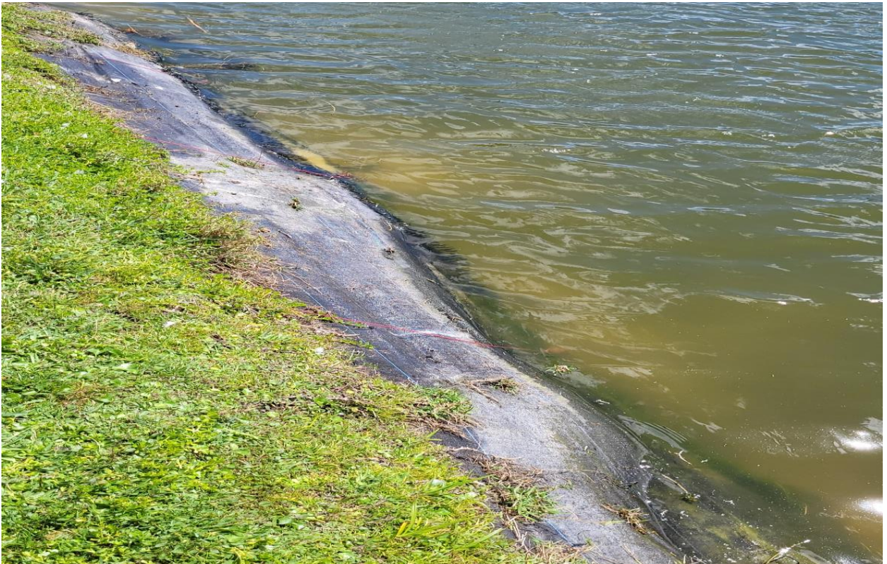
Photo 8: Completed re-installation of lake bank fabric material.
