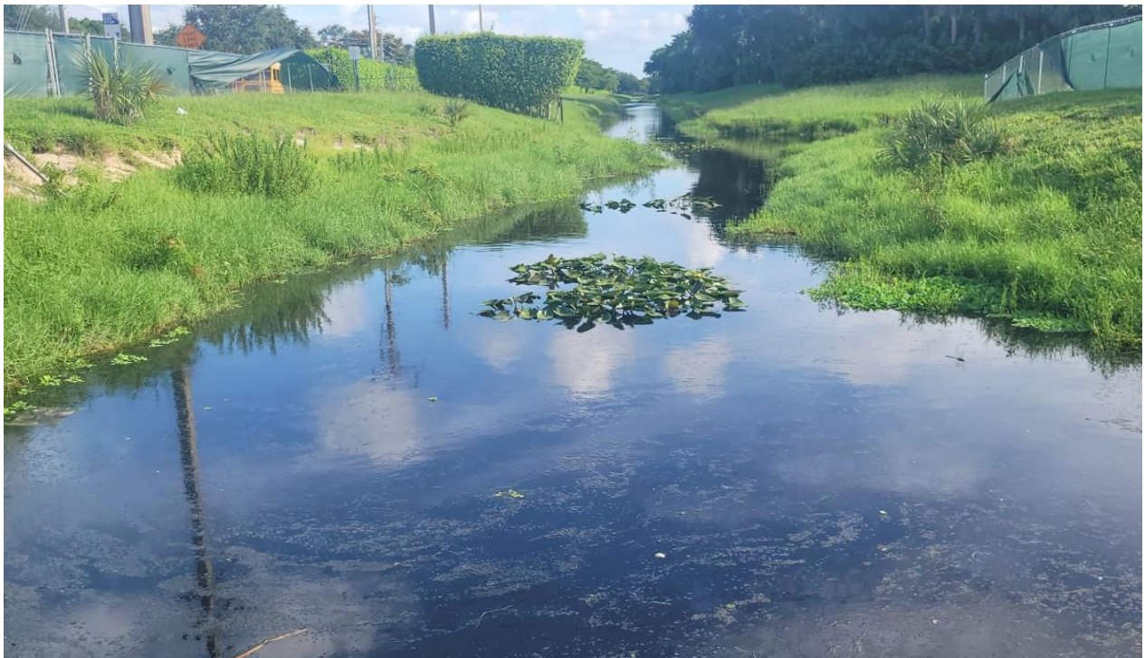
Photo 2: Canal bank erosion at Sheridan Street and N 72 Avenue, looking south.
