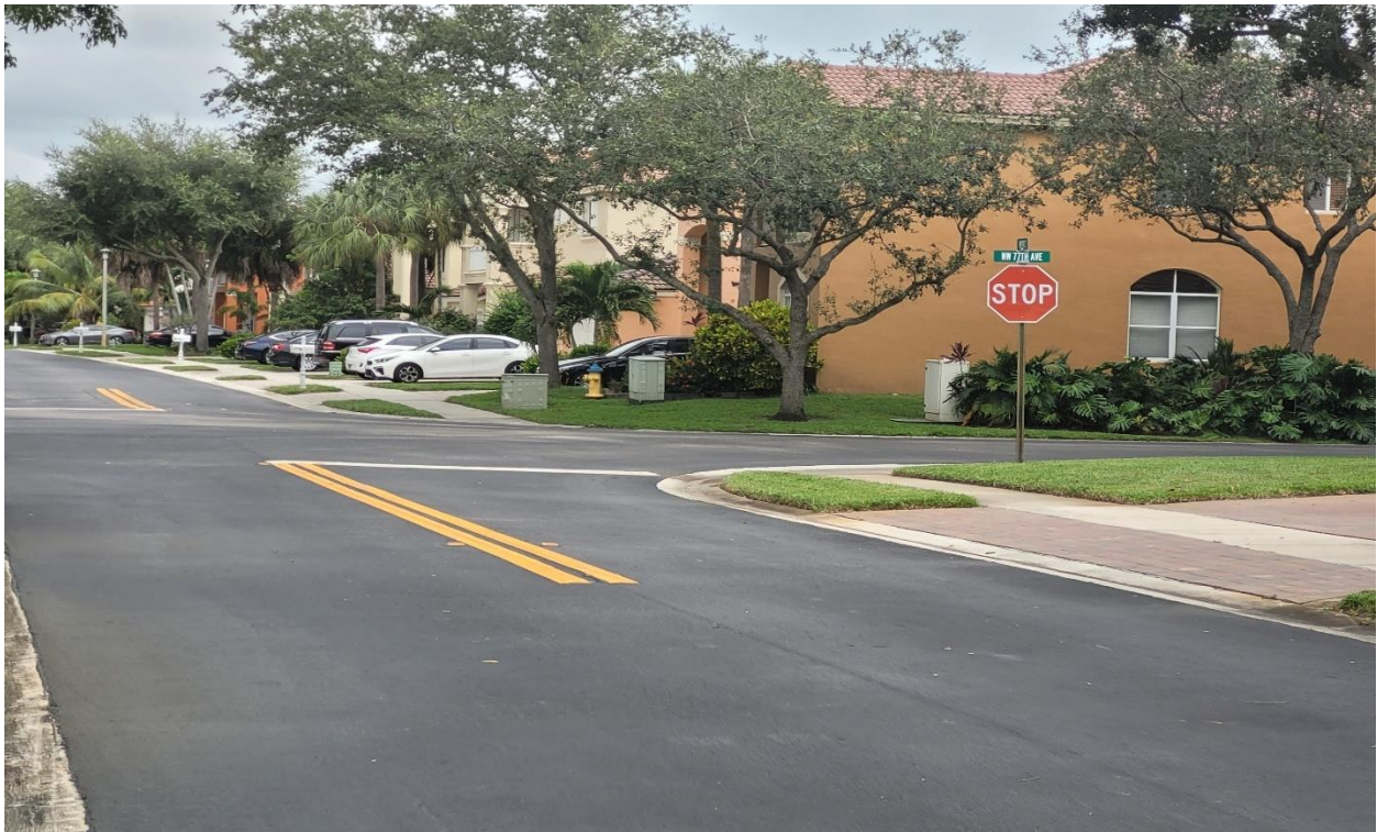
Photo 6: Sealcoating and restriping of internal WCCDD roads performed in 2022.
