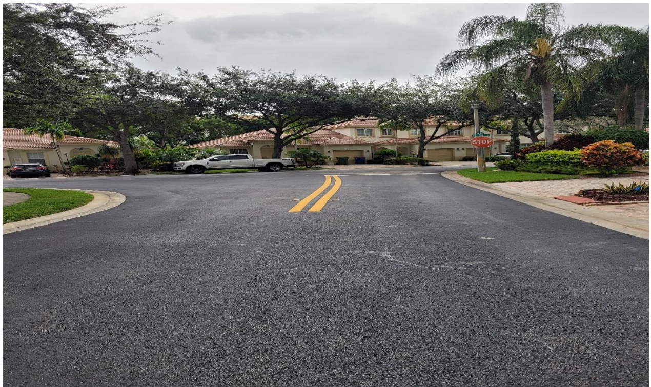
Photo 4: Sealcoating and restriping of internal WCCDD roads performed in 2022.
