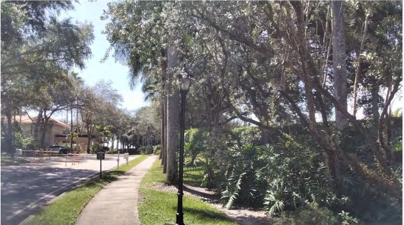
Above & Below: A light pole is in need of Clearance Pruning. The sidewalks and curbs and poles are in need of edging. Edging for the landscape beds and tree rings is also needed.
