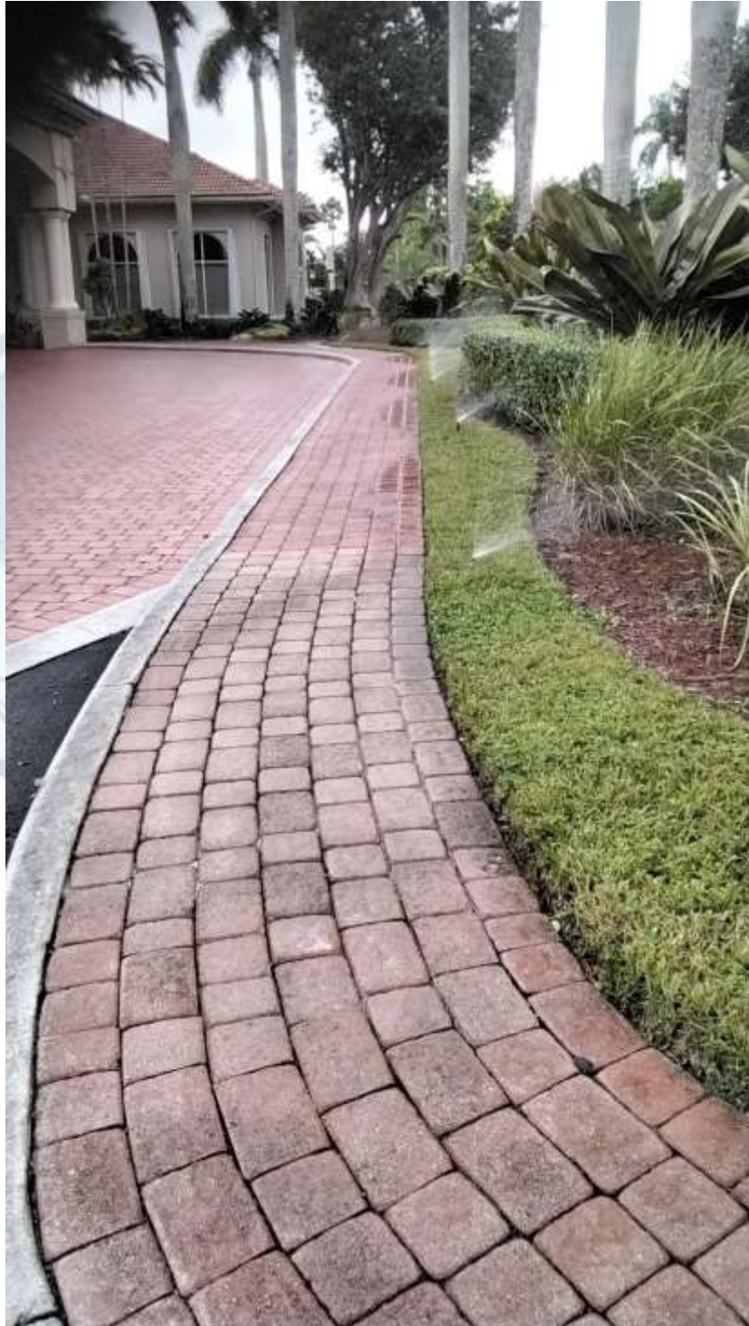
Above: Located at Clubhouse near Porte-cochere – This is Zone 4 on the location cock. A dry sidewalk is observed during operation. Pop-up heads are utilized in this area. Adequate pressure and coverage were observed for this high visibility area of the property.
