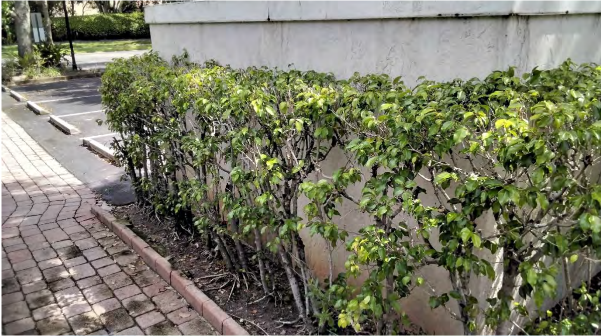
Above: The Ficus hedge material at the Clubhouse is aged and in poor condition. Narrow spaces need different species choices than in the past. Replacement with another plant type (possibly Podocarpus) is recommended.
