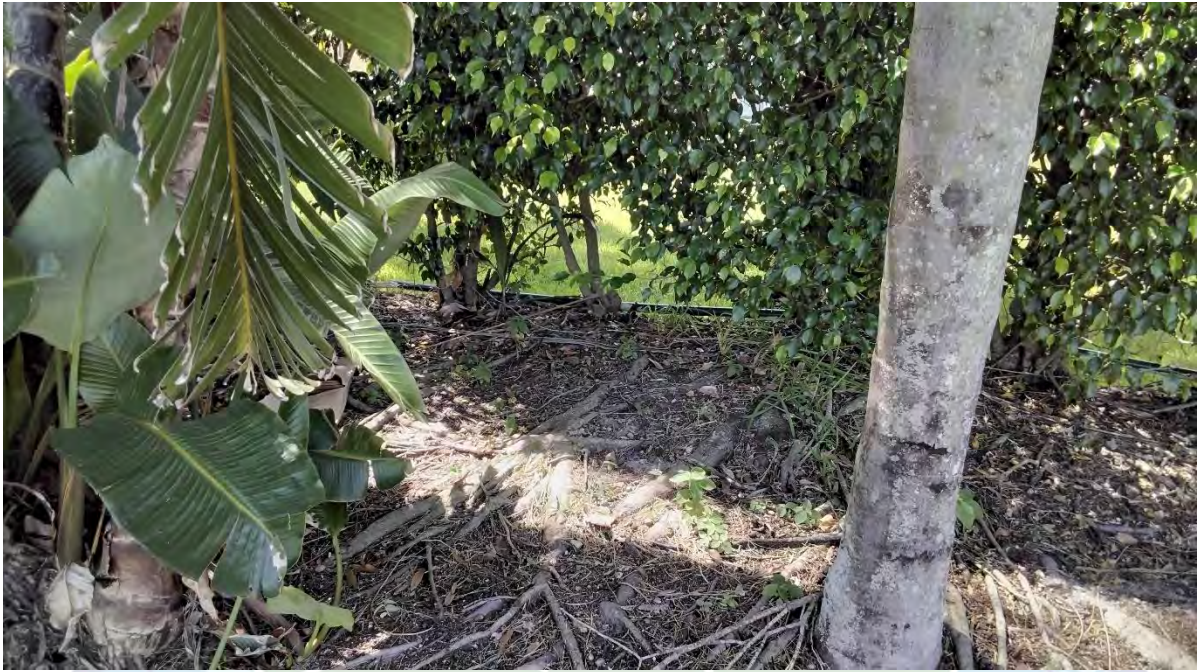
Above: Wires are shown running above ground and within the perimeter hedge. These wires can cause conflict with maintenance operations. Open areas in beds missing plants.
