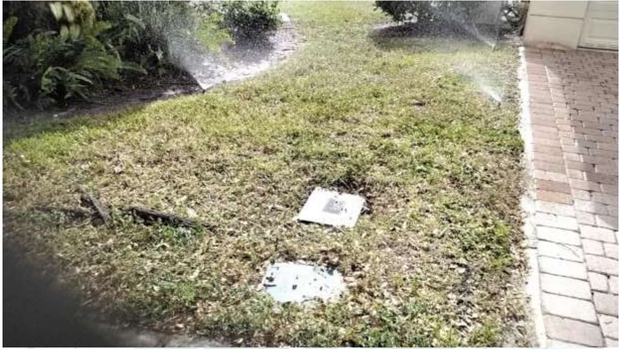
Above: Located within Mahogany Bend Community near 7390 NW 17 th Ct. This is Zone 20 on the location clock. Pop-ups and Risers are utilized. Coverage and pressure are adequate. Utility/Valve boxes are in need of edging.
