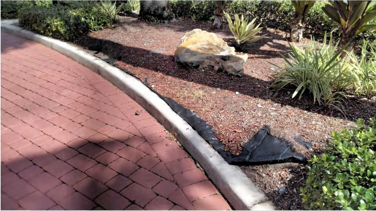
Above: Located near the fountain area – landscape liner material has rolled up and looks unsightly. Adding fresh mulch and securing this material will improve the appearance of this high visibility area.
