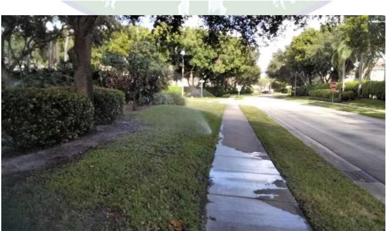
Above & Below: Located along the outer perimeter of the Clubhouse parking at the corner of NW 20 th St & N74 th Way – This is Zone 8 on the location clock. Rotors are shown along the sidewalk. Pressure was improved in this area and coverage was good.
