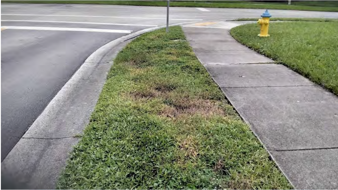
Above: Turf in the swale is in poor condition with dieback, weeds and discoloration.
