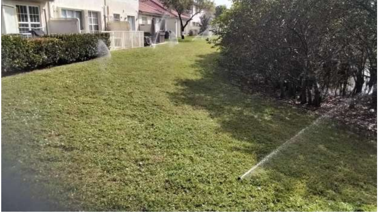
Above: Located within common area and along canal near NW78th Way. This is Zone 28 on the location clock. This is a large zone that utilizes rotors. Pressure is adequate and coverage is overlapping.
