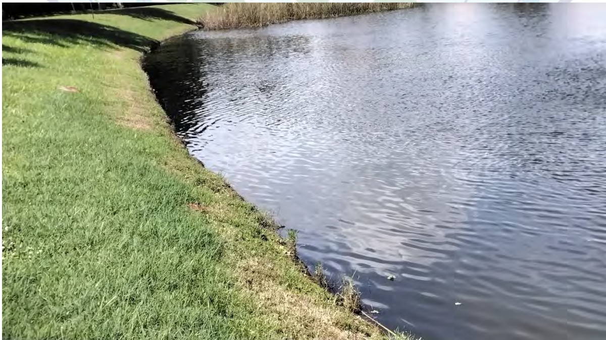
Above: There are signs of dieback for lawns along the lake edges, most likely due to string line trimmers cutting grass too short. Care must be taken not to scalp the turf in these areas.
