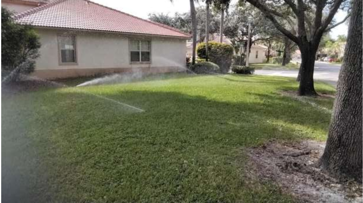
Above: Located in common area along NW 20 th St. This is Zone 11. Rotors and Pop-ups are utilized here. Good pressure and overlapping coverage are observed.
