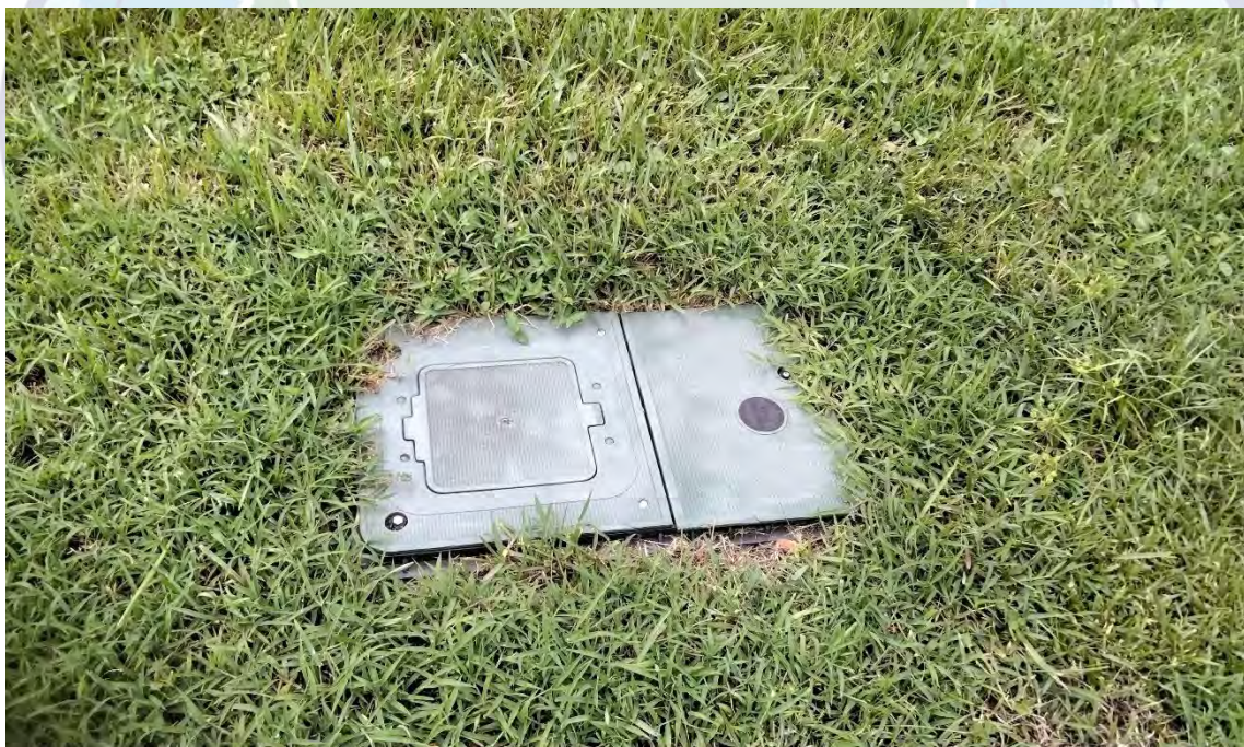
Above: A utility box is in need of edging. Edging of walkways, roads, curbs, sidewalks, hardscape features, landscape beds, tree rings, and utilities is typically required during each mowing service visit. The specifications for mowing, edging, turf weed control, need to be reviewed for what work met or did not meet specifications. The past contract had general services, or tasks, without performance standards for each that can be used to qualify work as complete or incomplete prior to making monthly payments.
