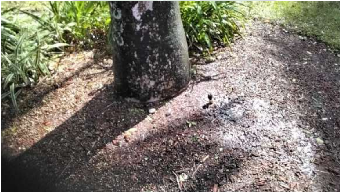
Above: Zone 6 at Clubhouse – A bubbler is in operation at the base of a Palm. As suggested by the Technician, this bubbler was to be capped as it was redundant within the landscape and was not necessary. There is adequate coverage by spray heads..
