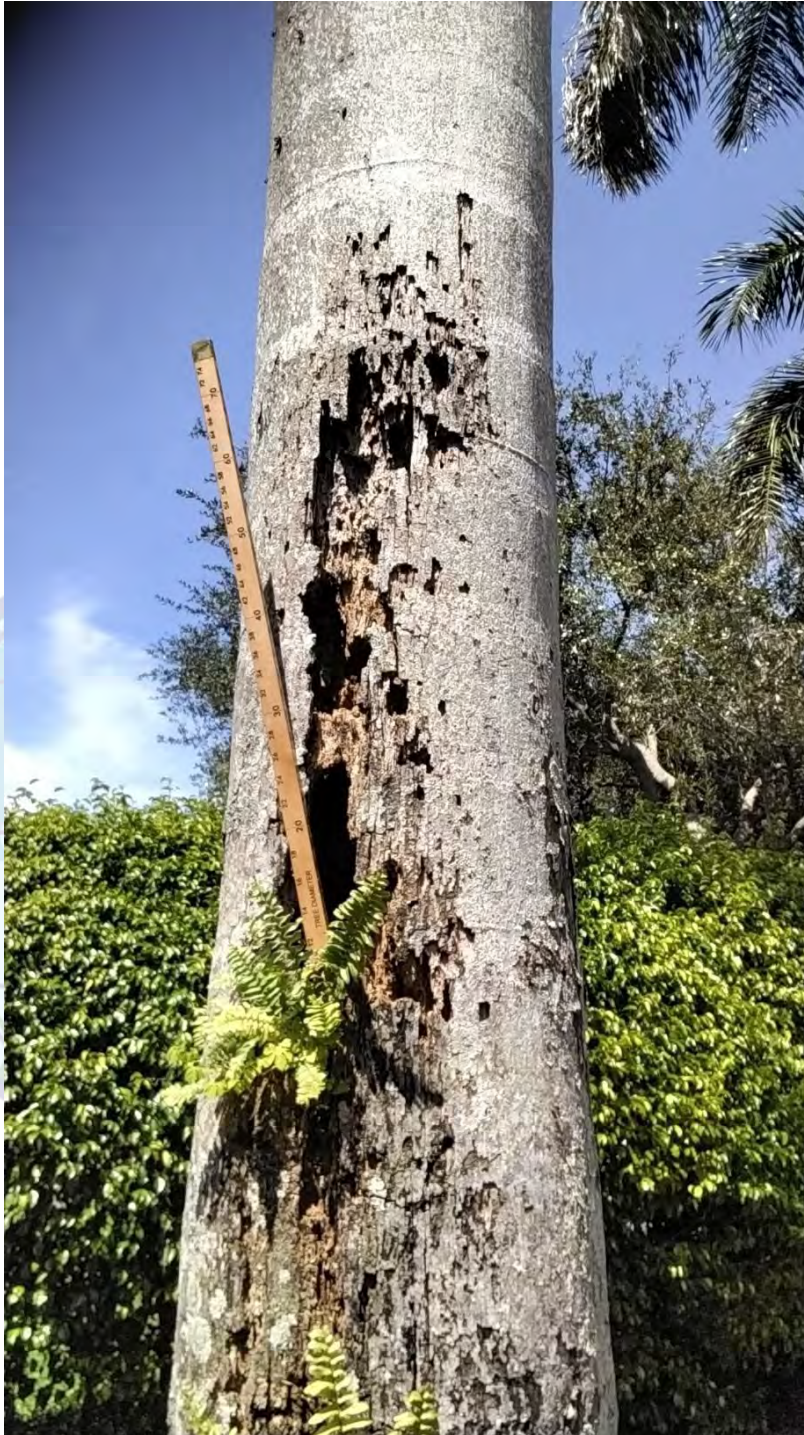
Above: Located on Southbound NW 76 th Ave. A badly decayed and hollow Royal Palm trunk is shown. A separate Arborist Report can be provided to facilitate removal.
