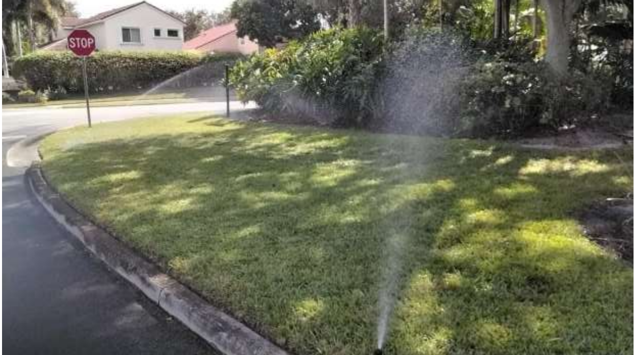
Above: Located near Clubhouse exit along NW 20 th St – This is Zone 9 on the location clock. A mix of Rotors, Pop-ups and Risers are shown. Good pressure and coverage is displayed next to a dry street.
