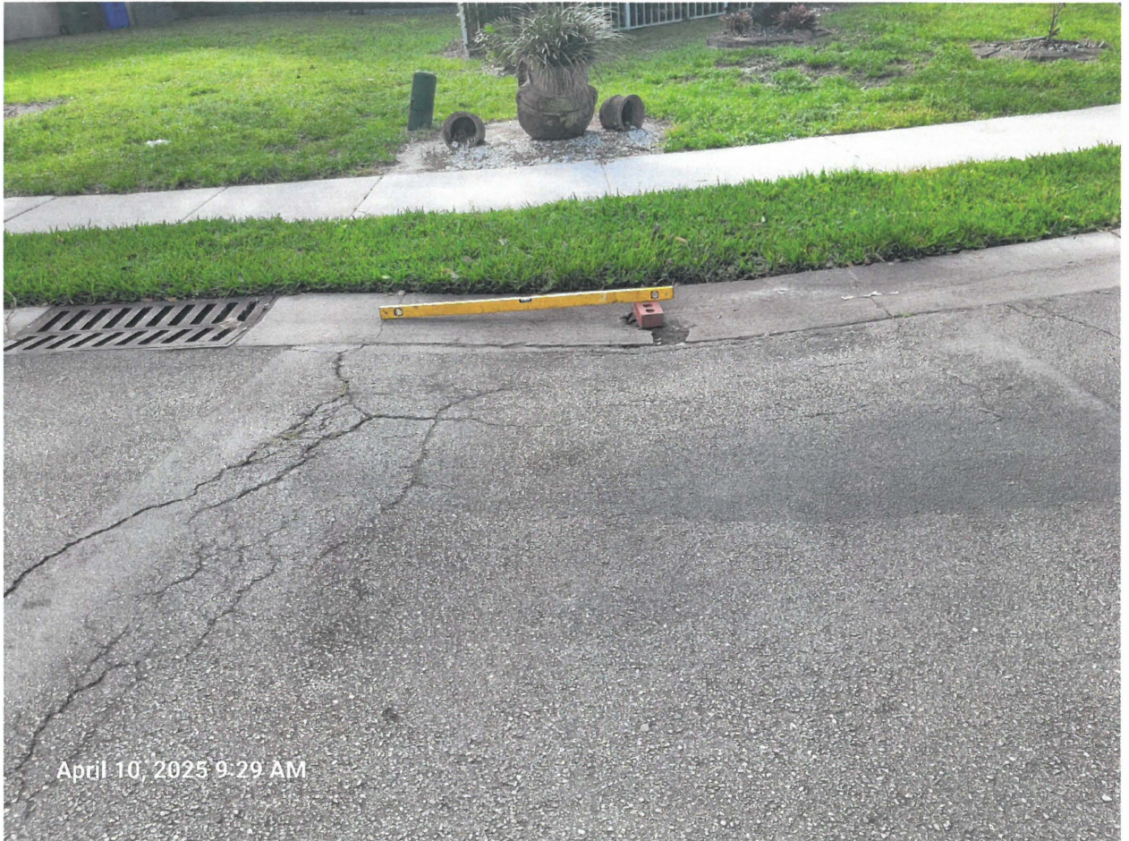
Photo No. 1: Approximately 2-inch settlement adjacent to stormwater structure NW 19 th Drive and NW 75 th Way
