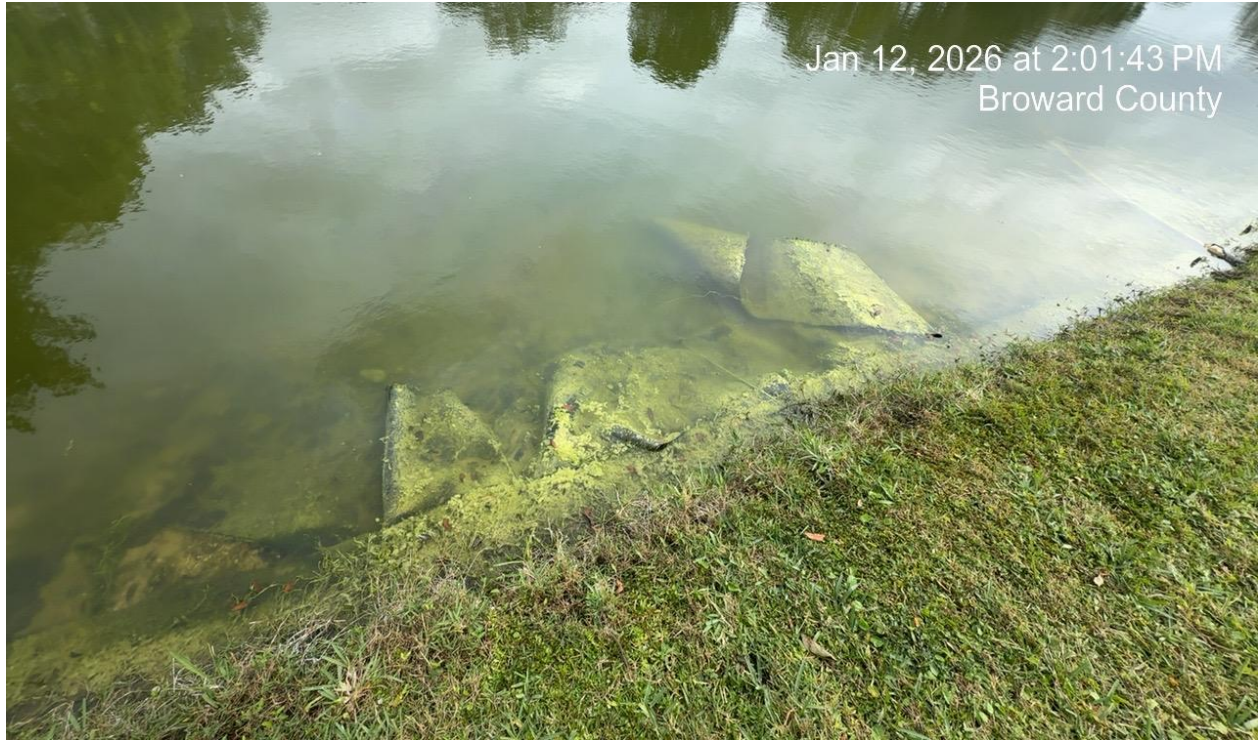
Photo 3: Lake 9 deteriorated geo fabric textile material detached from support bag.
