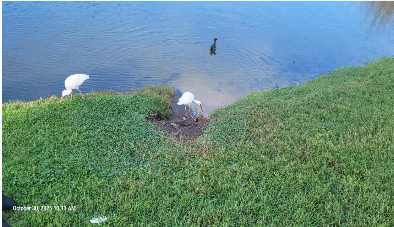
Photo 1: Lake 6 wash-out at base of bank. Birds foraging within area of concern.
