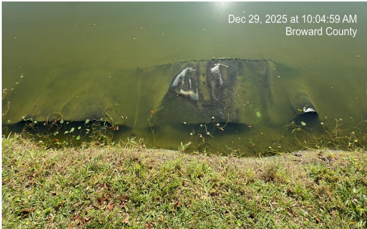
Photo 1: Lake 2 deteriorated geo fabric textile material.
