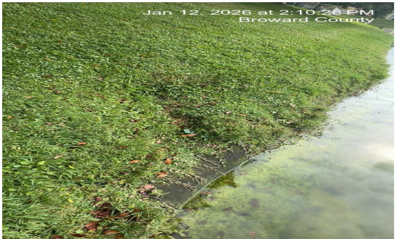
Photo 4: Lake 9 deteriorated geo fabric textile material and bank erosion/ depression.
